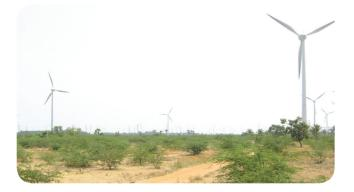
This project is a 36 MW grid connected wind farm. It generates renewable energy using 45 Enercon Wind Energy Generators at 800 KW each. The power generated is fed into the local grid and is also sold for captive use.
